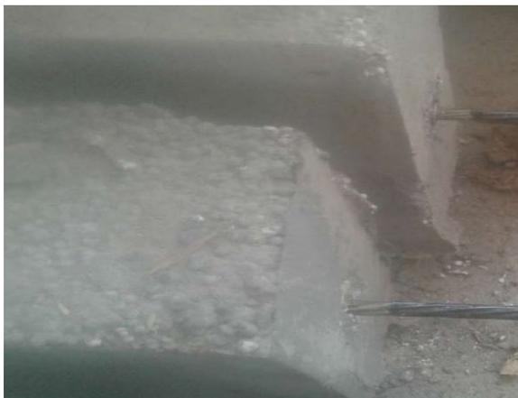
Fig. 10. Elongation after tensioning the tendon
