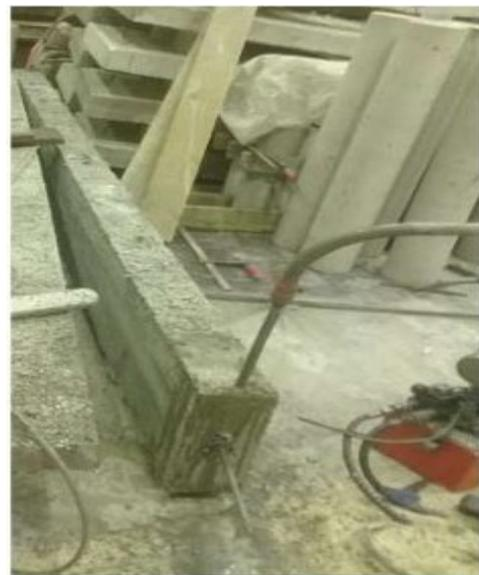
Fig. 12. Grouting injection
